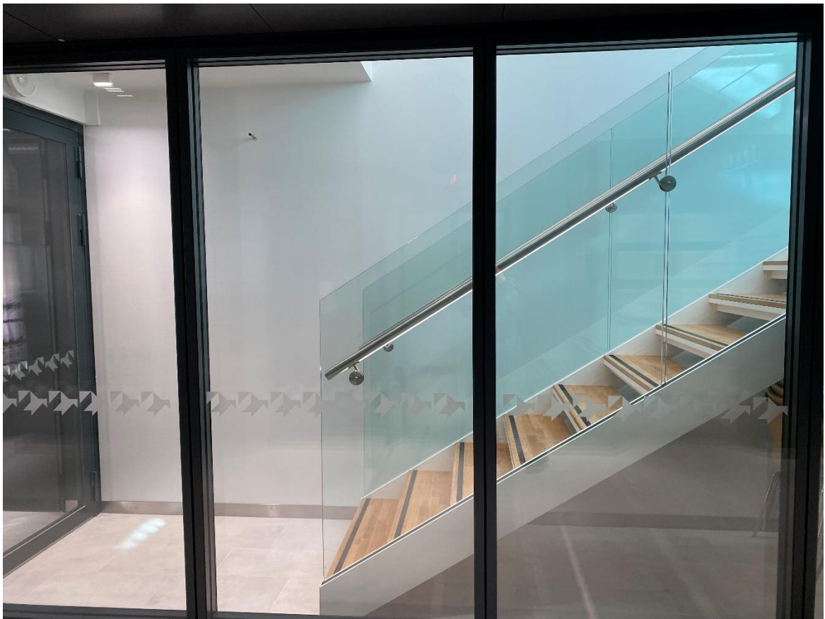
3. White painted walls surrounding a staircase on the same floor (four photos)
