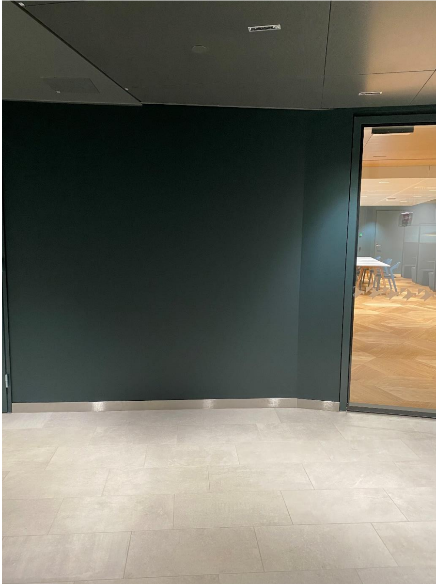
2. Black painted wall on the same floor
